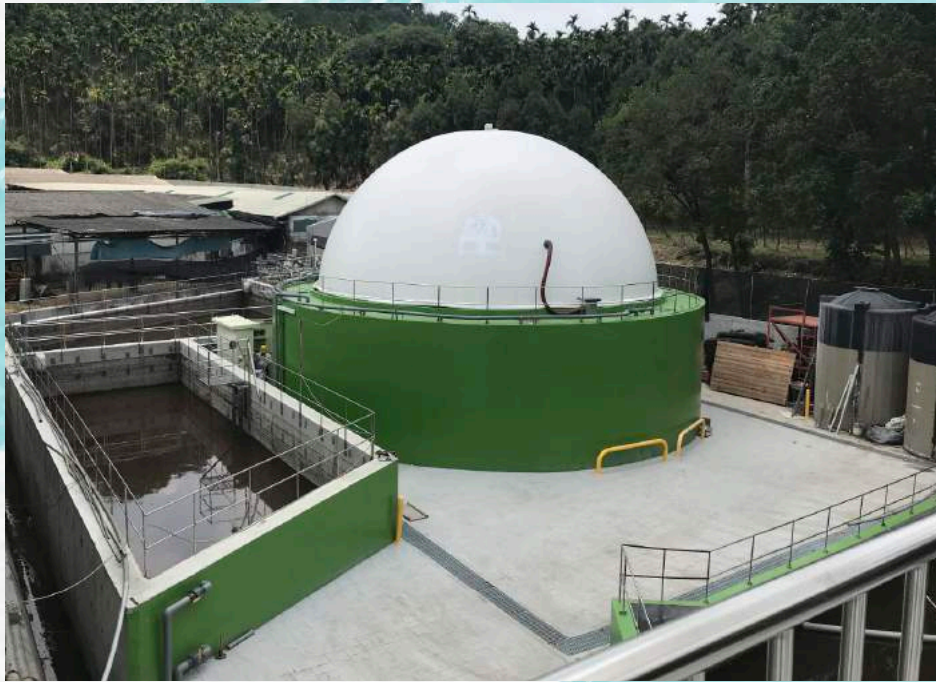
Taiwan's first two-stage anaerobic pig farm biogas plant.
