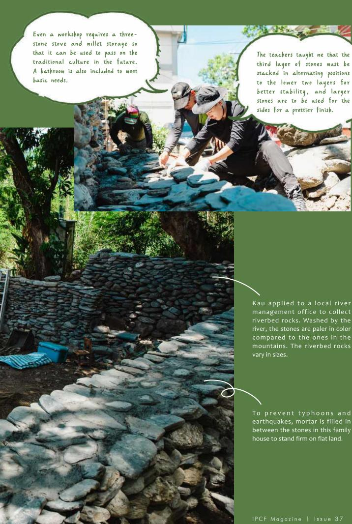
To prevent typhoons and earthquakes, mortar is filled in between the stones in this family
